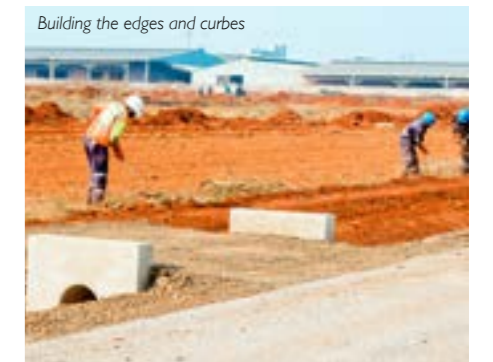
Building the edges and curbes
